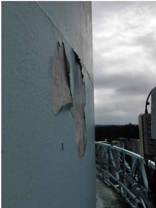
Tank Exterior Coatings
