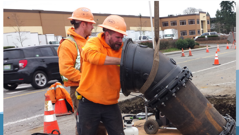
Contactors lower 20-inch pipe for water main installation.
