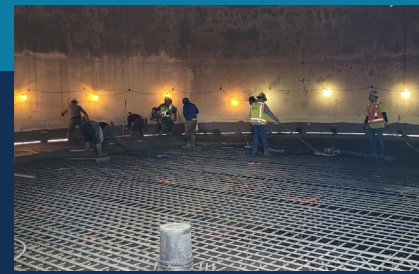
Installing Concrete at the Steilacoom Boulevard Tank Seismic Retrofit Project
