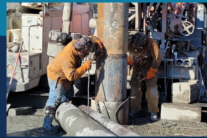
Installing Well Casing at R-2 Well
