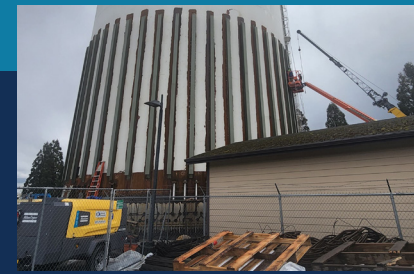
Steilacoom Boulevard Tank Seismic Retrofit Project
