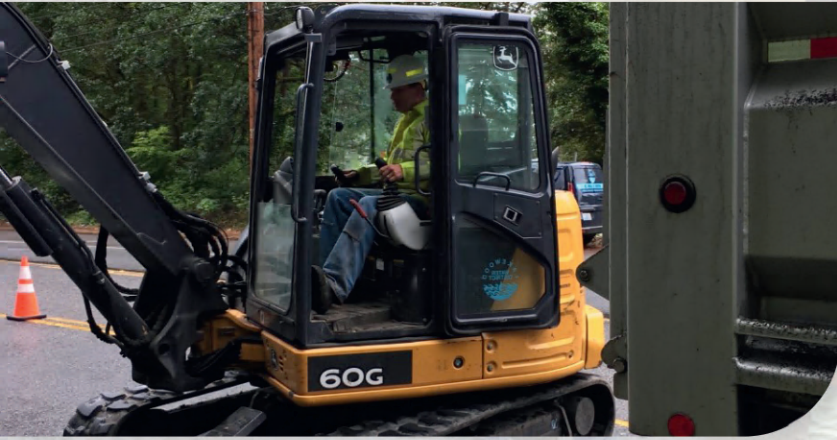
(Above) Eric uses a mini-excavator to load spoils into a dump truck
