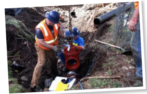
Sam and Shaun install an 8-inch gate valve off Chicago Avenue
