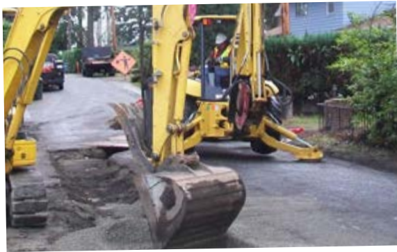
Construction on Langlow Street, off Veterans Drive SW
