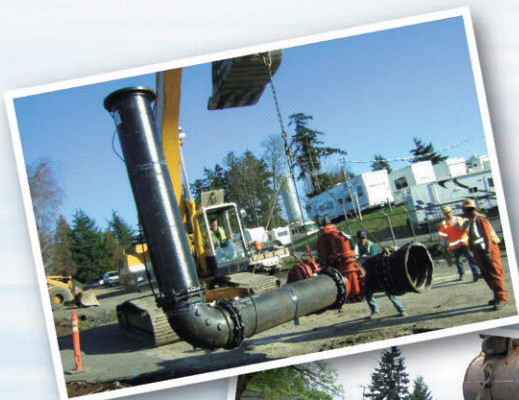
Wholesale Transmission Main installation.
