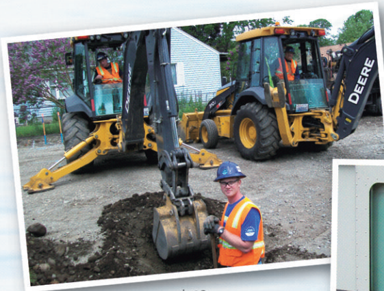
Installing new water services.
