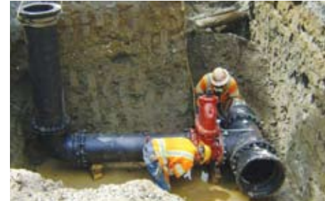
Crews installing 20" pipe
