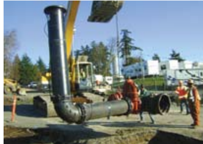
Crews installing 20" pipe
