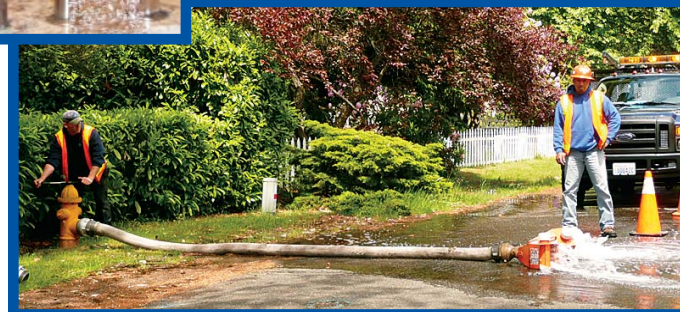
Flushing a nearby neighborhood street
