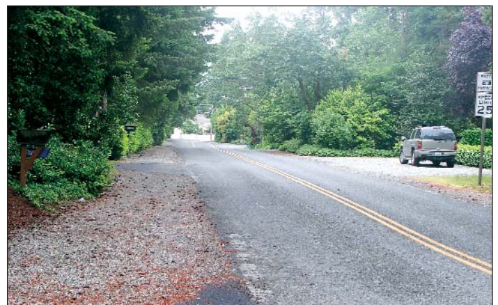
A view of Interlaaken Drive after completion of the pipe replacement project.
