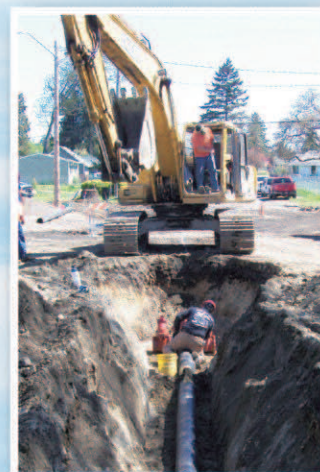
New 8-inch ductile iron pipe replaces old 4-inch asbestos concrete pipe.
