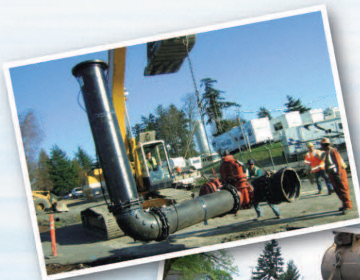
Wholesale Transmission Main installation.
