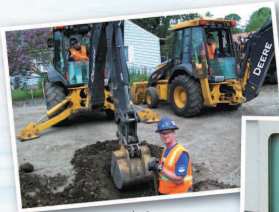
Installing new water services.
