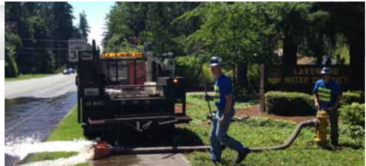
Lakewood staff conducting annual flushing of water mains.
