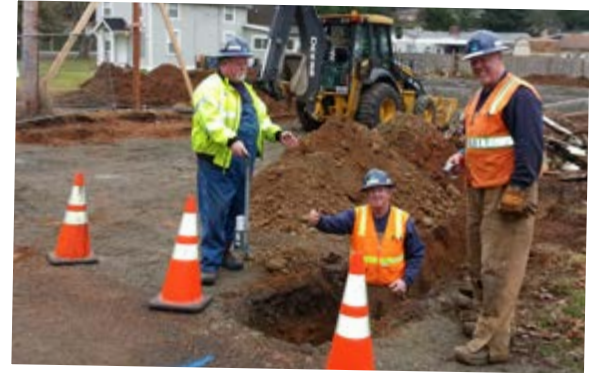
Dick, Rich, and Sam install a new water service line for a customer on Wildwood Avenue
