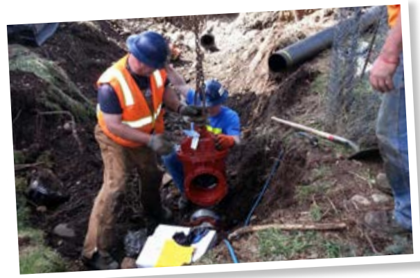
Sam and Shaun install an 8-inch gate valve off Chicago Avenue
