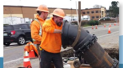
Contactors lower 20-inch pipe for water main installation
