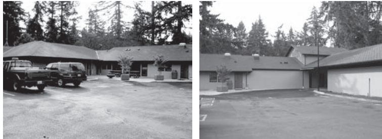
The District's new Shop and Office Remodel & Addition
