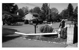
up around the inside of the 4-inch and larger water mains. There are no health risks associated with these deposits. We perform high-velocity flushing of our system, pulling water from a storage tank or reservoir, then proceeding from hydrant to hydrant, turning them on full speed out of the front pumper port. This action causes
