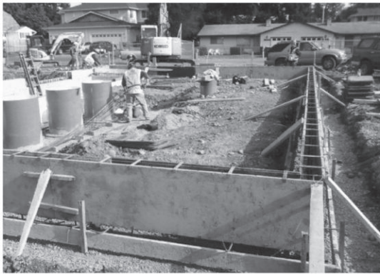
Under construction in mid-May.
