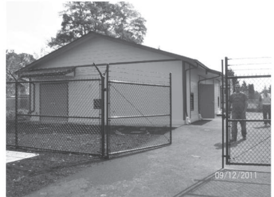
Completed Booster Station.
