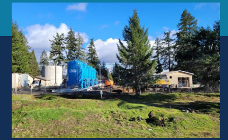
Scotts Wellfield Treatment Project
