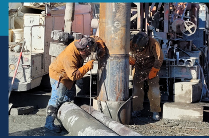
Installing Well Casing at R-2 Well
