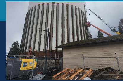
Steilacoom Boulevard Tank Seismic Retrofit Project
