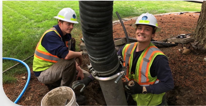
(Above) Kyle and Tyler use rented vac truck to free meter boxes of tree roots without having to remove trees
