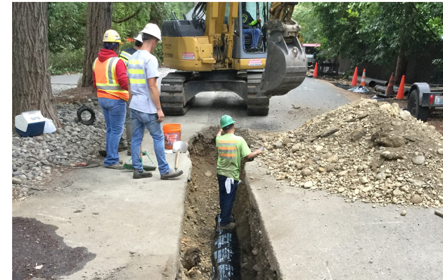
Lake Steilacoom Drive project
