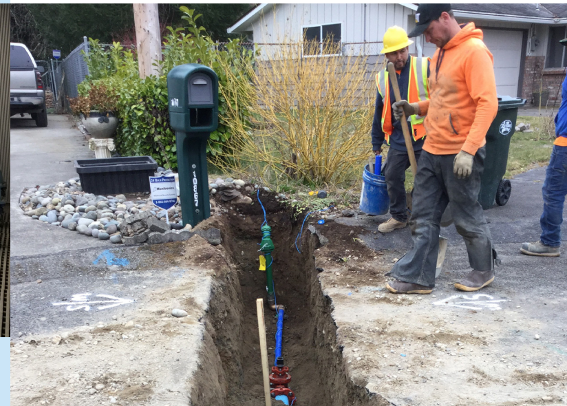
Arrowhead Phase 2 old pipe replacement
