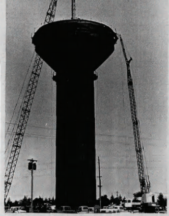
Paint Job Is Next
