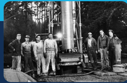
Drilling a Well on Hipkins Road, 1952
