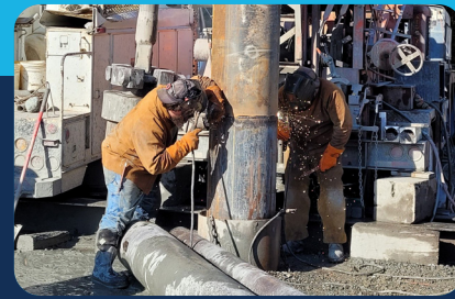
Well Casing 112th St R-2 Well
