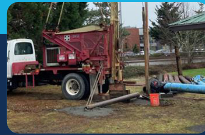
P-1R Well Rehabilitation at Steilacoom Blvd
