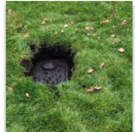
*Photo is a water meter that had to be cleared from under sod/grass.
