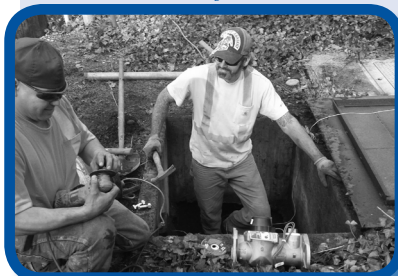
Pape & Sons installs 3-inch meter for Dower Elementary School.
