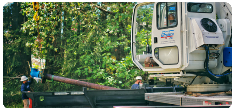
(Above) Turbine pumps, motors, valve at WTM Booster Station (Bottom) PumpTech removes well pump & motor
