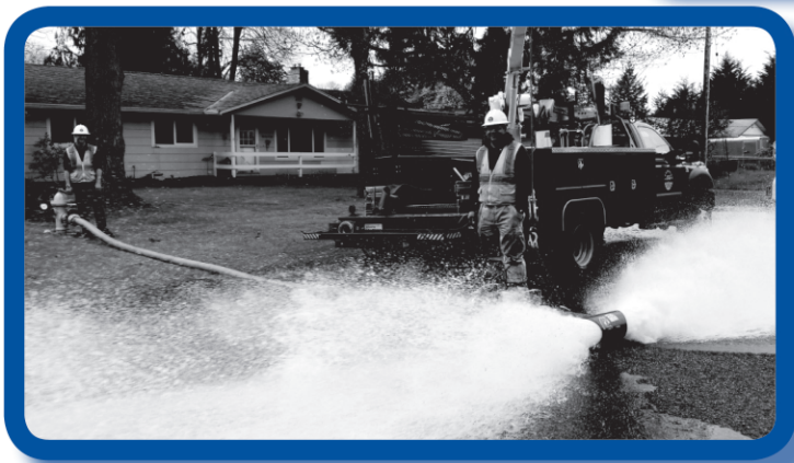
Ryan and Seth flushing your water mains to help ensure the highest water quality.
