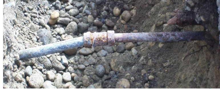
Repaired sewer service project
