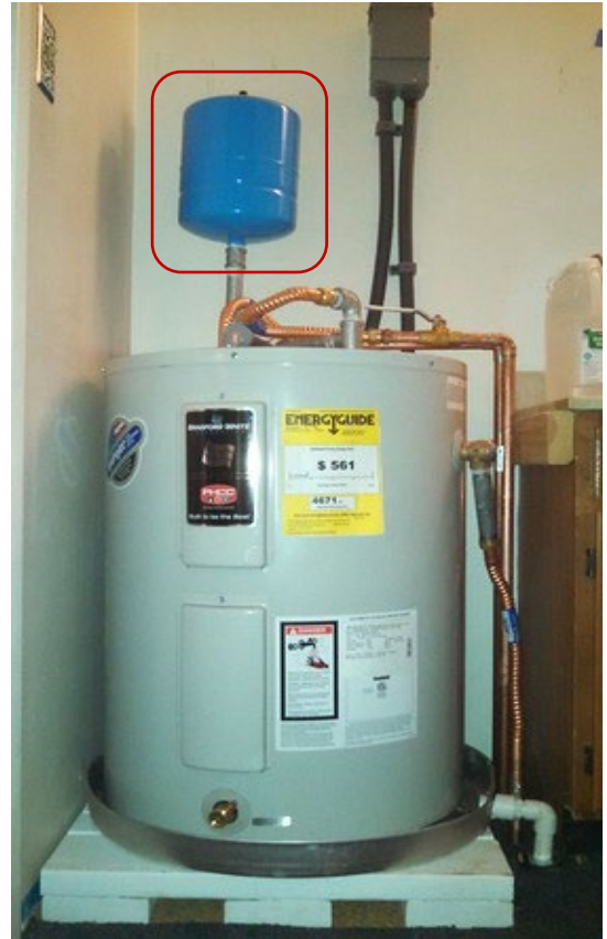
Typical Hot Water Expansion Tank Installation
