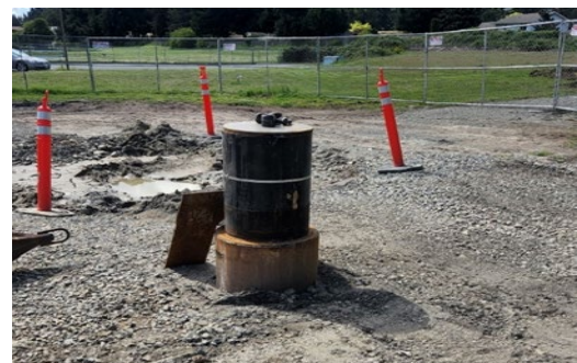
Completed R-2 Wellhead
