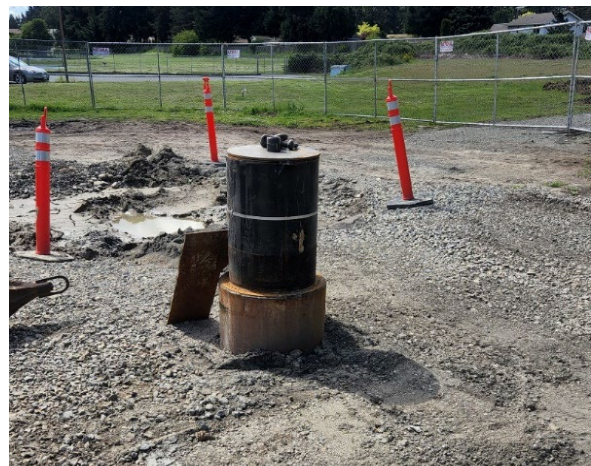
Completed R-2 Wellhead
