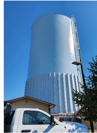
Tank with shell stiffeners around exterior; with intermediate and topcoat in progress, with topcoat nearly complete (Left to Right).
