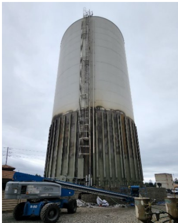
Tank with shell stiffeners around exterior; with intermediate and topcoat in progress, with topcoat nearly complete (Left to Right).
