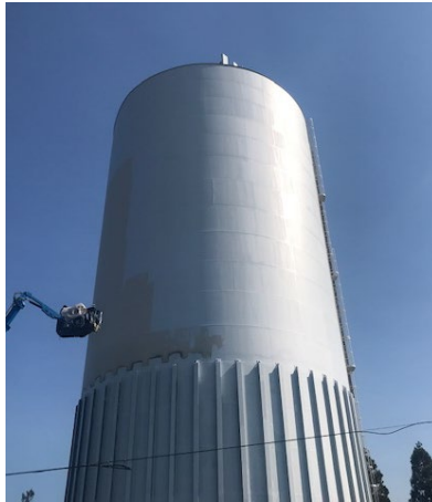
Tank with shell stiffeners around exterior; with intermediate and topcoat in progress, with topcoat nearly complete (Left to Right).
