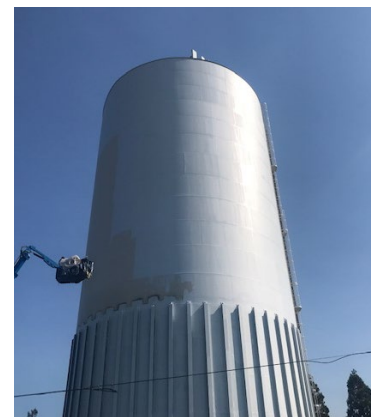
Tank with shell stiffeners around exterior; with primer in progress; with intermediate coat in progress (Left to Right).
