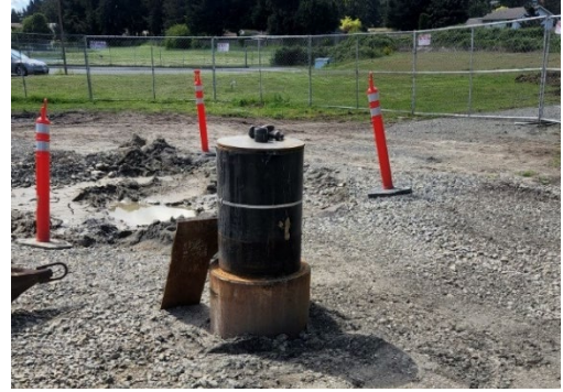
Completed R-2 Wellhead
