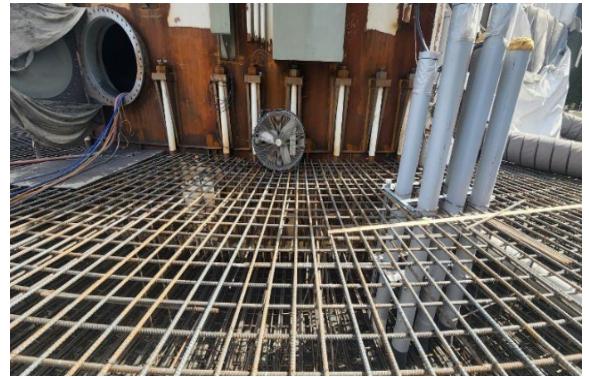
Foundation rebar on tank exterior.
