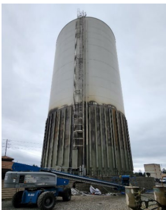
Tank with shell stiffeners around exterior; with primer in progress; with intermediate coat in progress (Left to Right).
