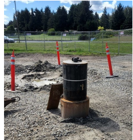
Completed R-2 Wellhead
