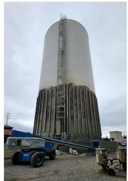
Tank exterior with exterior primer in progress.
