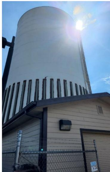
Tank exterior with shell Stiffeners around exterior.
