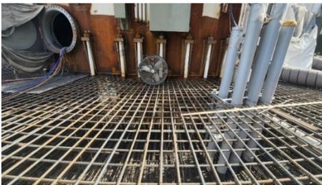
Foundation rebar on tank exterior.
