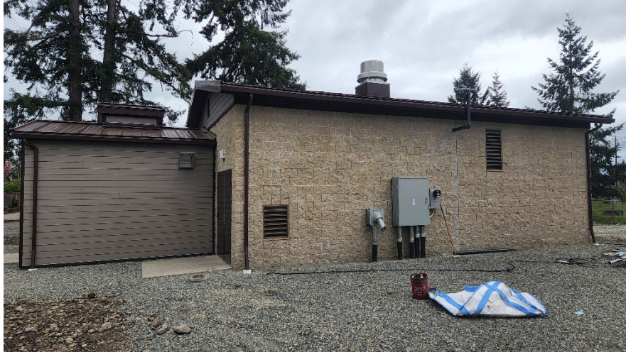
G-3 Well Building Exterior (Well and Pump on Left, Treatment and Electrical on Right)
