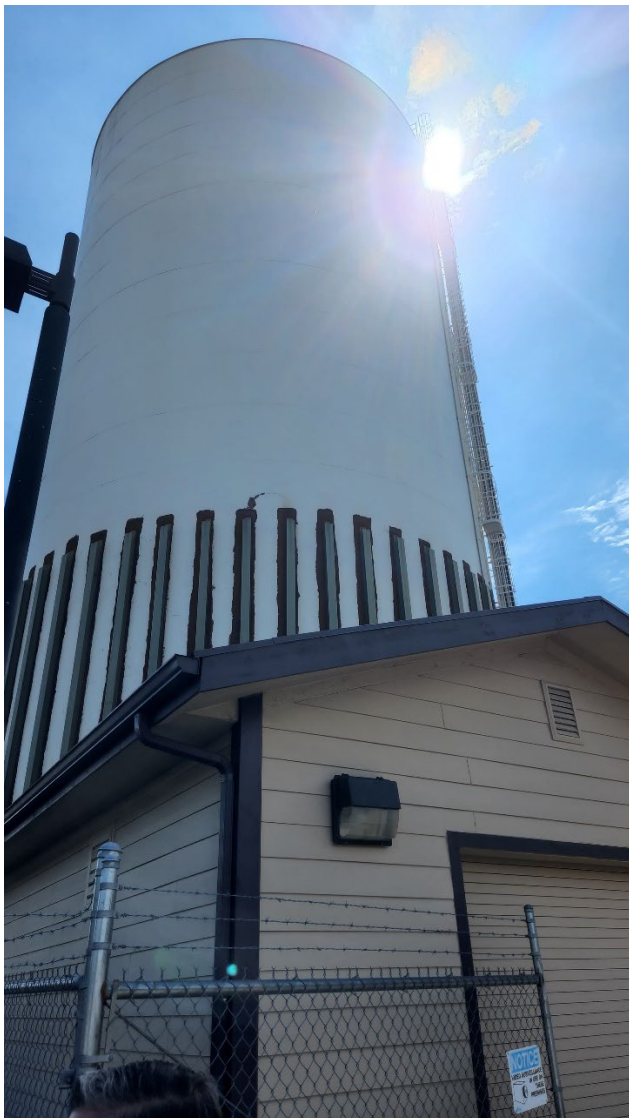
Tank exterior with shell stiffeners around exterior.
