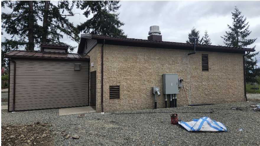
G-3 Well Building Exterior (Well and Pump on Left, Treatment and Electrical on Right)
