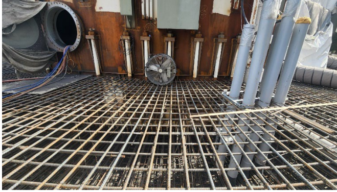
Foundation rebar on tank exterior.
