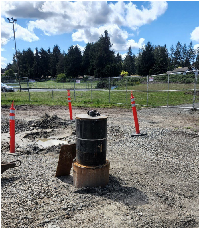
Completed R-2 Wellhead
