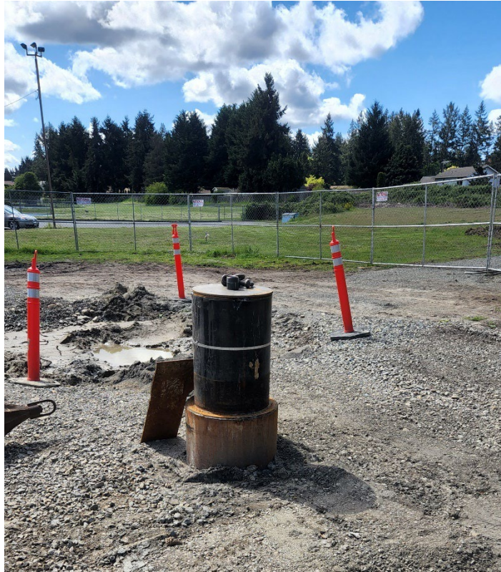
Completed R-2 Wellhead
