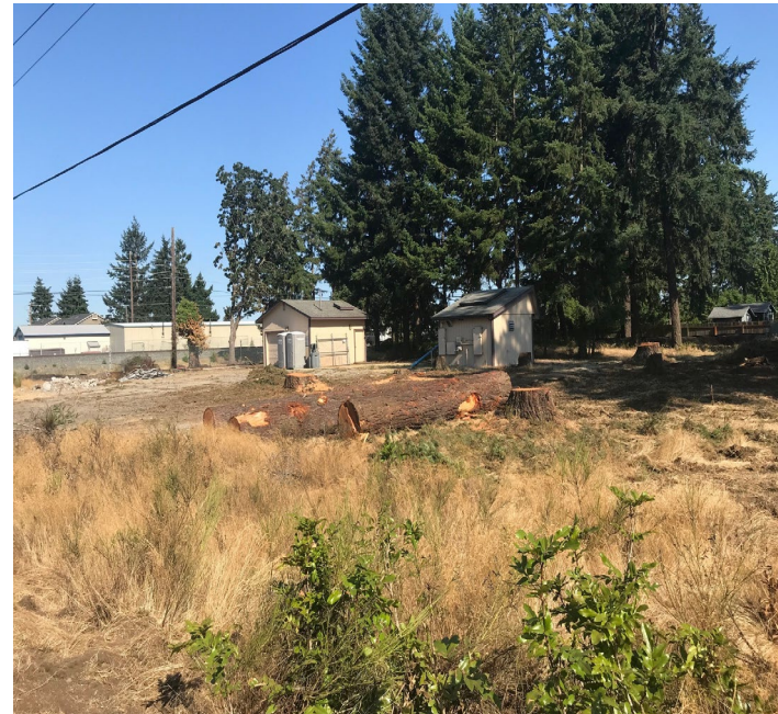
Clearing the property
