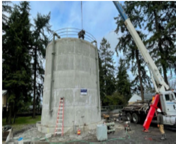
Setting top rail and overflow Pipes on GAC Backwash tank
