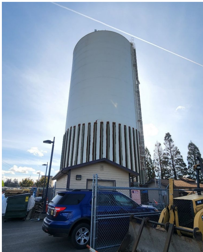
Tank exterior with shell stiffeners around exterior.
