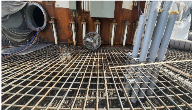
Foundation rebar on tank exterior.
