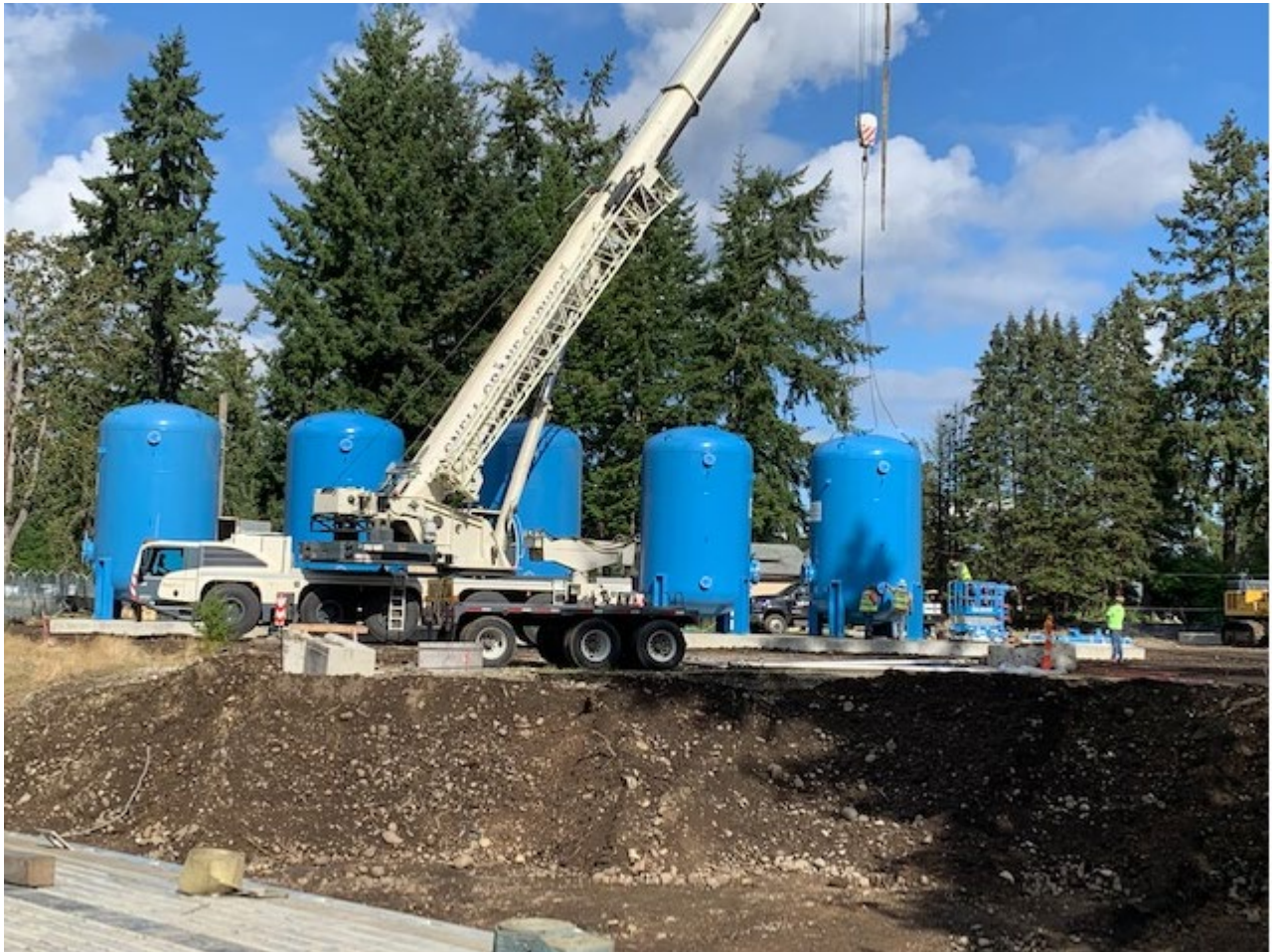
Photo: GAC filters being placed on their foundation
