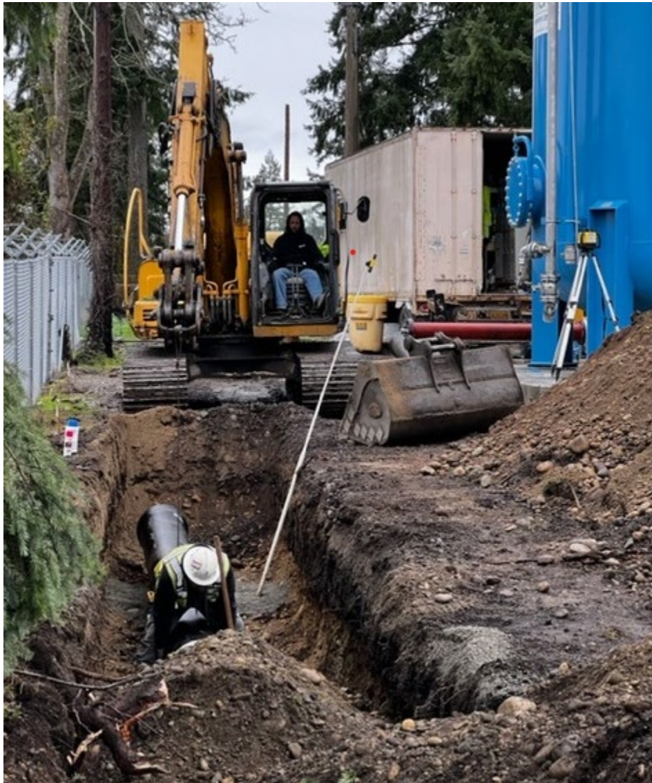
Photo: Yard piping for G-1 and G-2 Wells being installed
