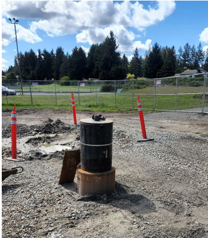
Completed R-2 Wellhead
