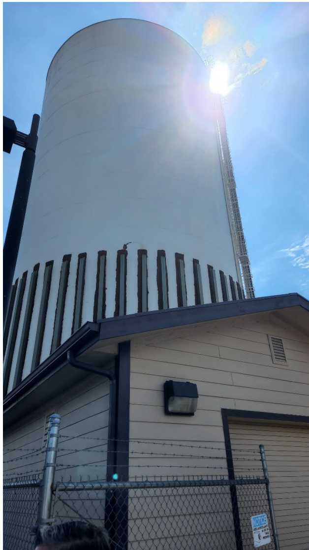
Tank exterior with shell stiffeners around exterior.
