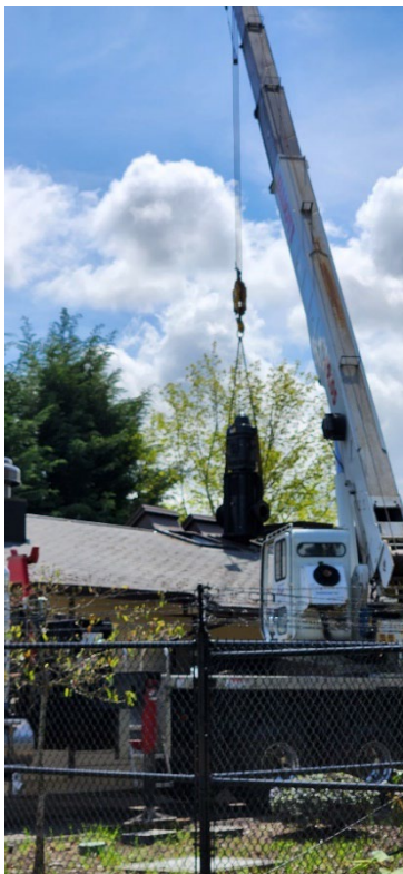
Crane lifting pump for service
